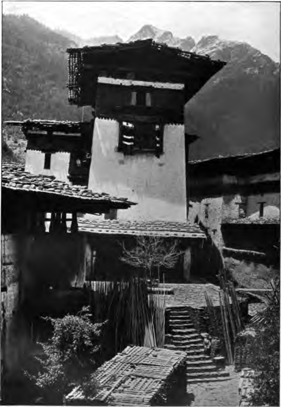
INTERIOR OF DUG-GYE-JONG
